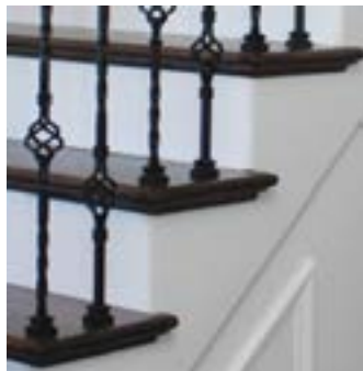
Open Tread Stairway
